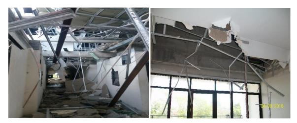
Fig. 4 – Example of architectural damage caused by the earthquake: Ceiling damage due to the falling of the material above it at the rental low-cost housing flats
