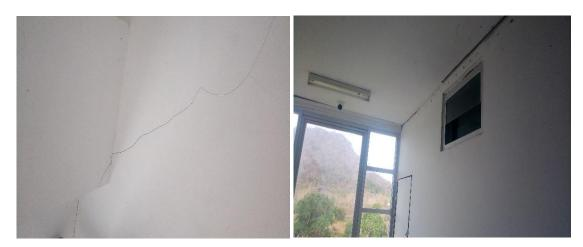
Fig. 5 – Example of minor damage caused by the earthquake: Hairline Cracks on the wall and falling of ceiling list at Sumbawa Technology University flats
