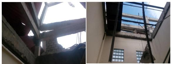
Fig. 3 – Example of major damage to structure caused by the earthquake: Crushing at beamcolumn joints at the North Lombok Police Station housing flat
