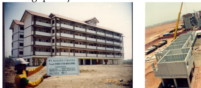
Gambar 8 Sistem Waffle Crete
