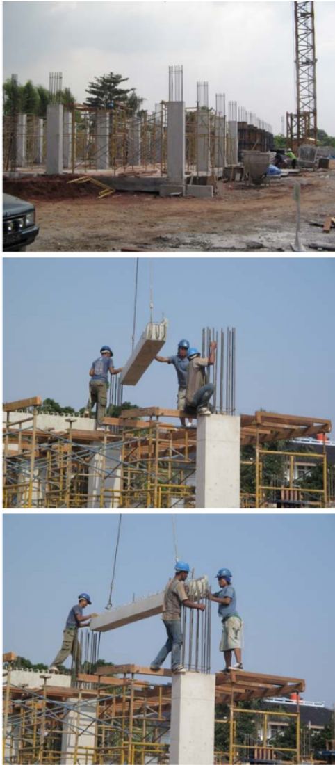
Fig. 1. Erection process the precast system.
