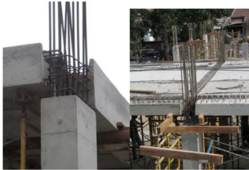
Fig. 2. Joint on the beam (the precast system).
