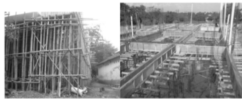
Fig. 3. Conventional system using wood for formwork and scaffolding.
