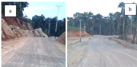
Fig. 5. New Road work results and 100% physical progress
