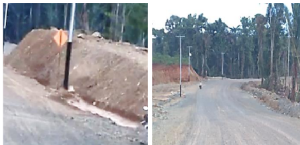
Fig. 9. Waterways (Drainage) on New Roads and physical progress, 20%
