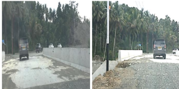
Fig. 7. The results of the bridge work and 100% physical progress
