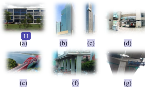
Fig. 16: Implementation examples of base isolation in Indonesia: (a) Office of PUPR Padang (2010); (b) Gudang Garam Office (2013); (c) Thamrin Nine (2020); (d) Office of Wijaya Karya (2018); (e) Holtekamp Bridge (2020); (f) LRT Jabodetabek (2019); (g) Pettarani toll road (2021).
