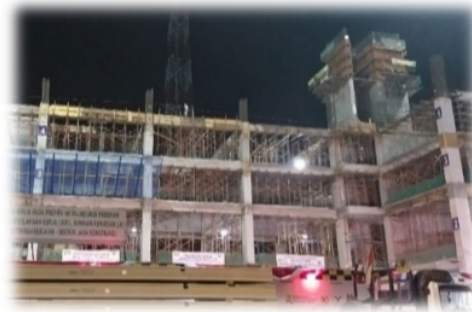
Construction phase of building
