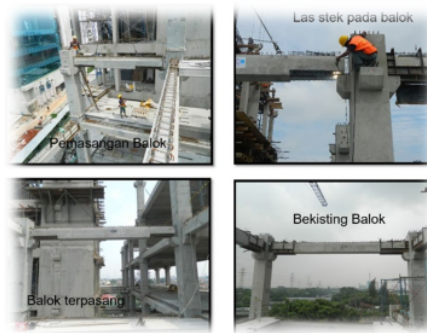
Construction phase of building
