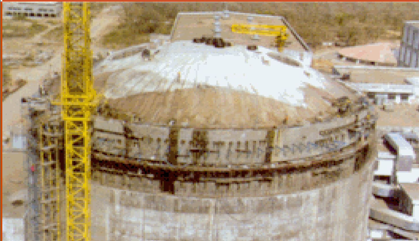
IC Dome after completion of concreting
