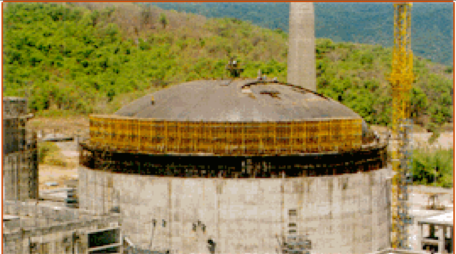
Soffit formwork of IC dome
