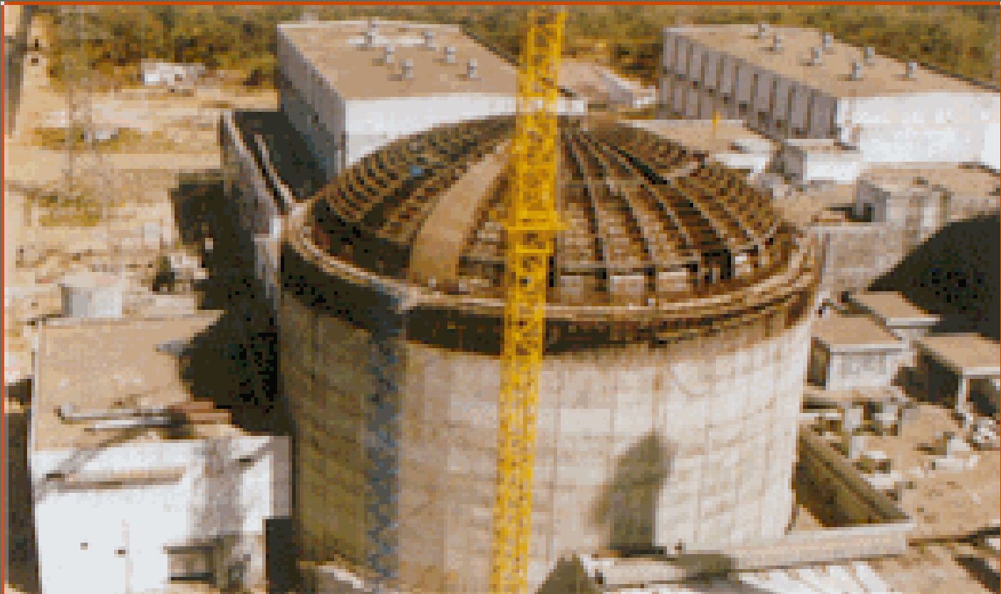
IC dome supporting structure in position
