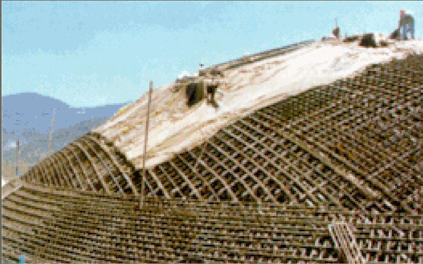
Reinforcement layout of IC dome
