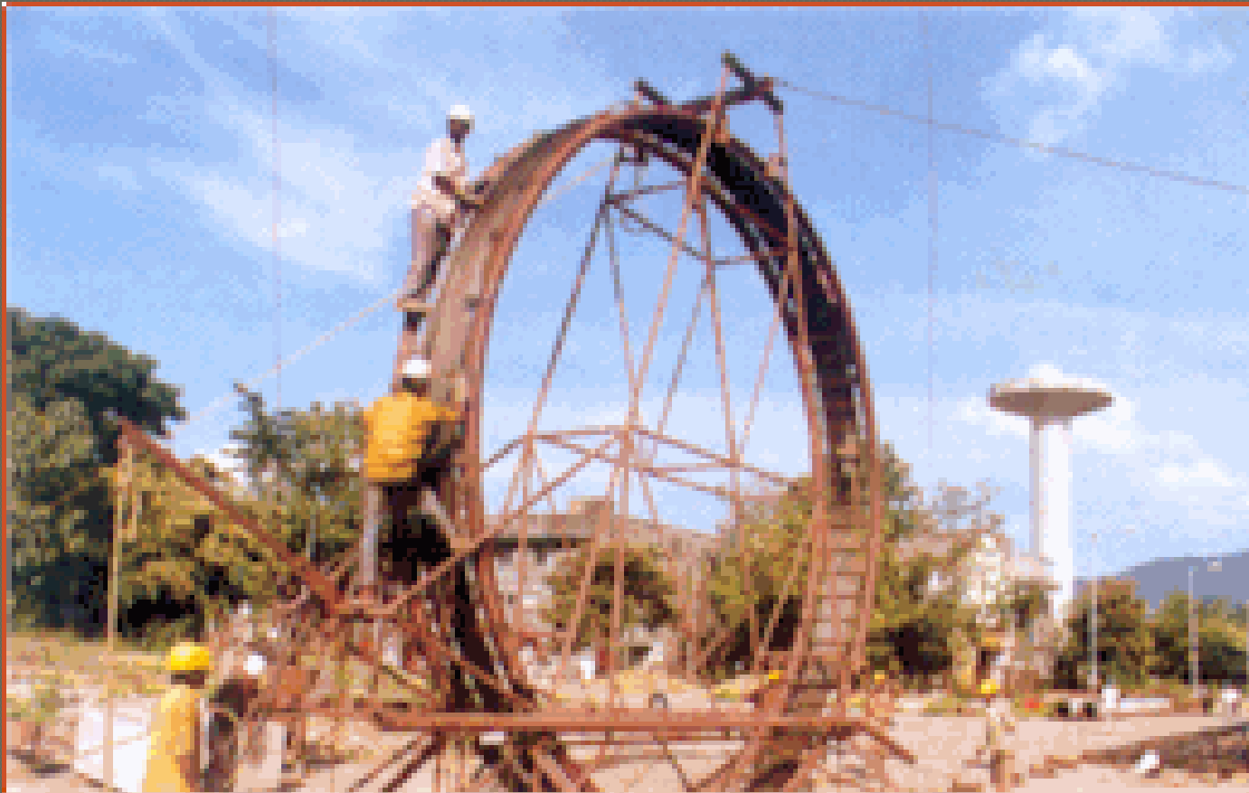
Decoilers used for erection of pre-stressing cables
