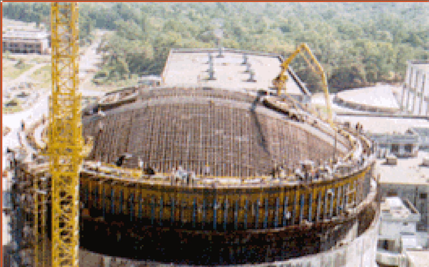
Pre-stressing cable layout of IC dome
