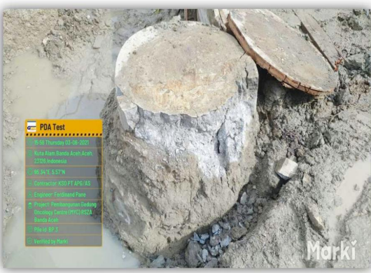
Pile Name : BP.3 Date of Testing : June 03 rd , 2021
