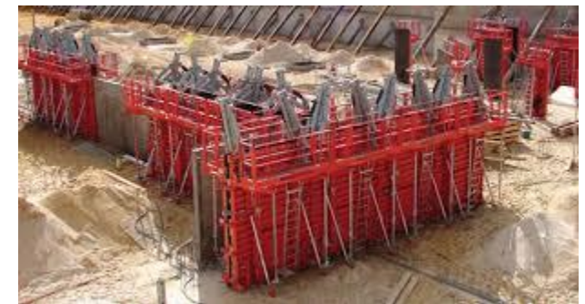
Sistem Formwork Bearing Wall
