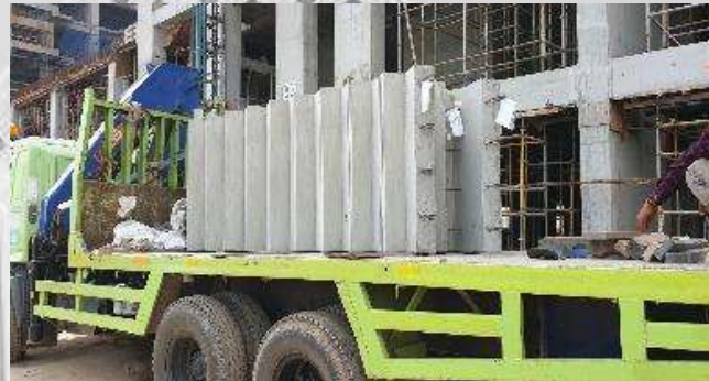
Precast Stair Case
