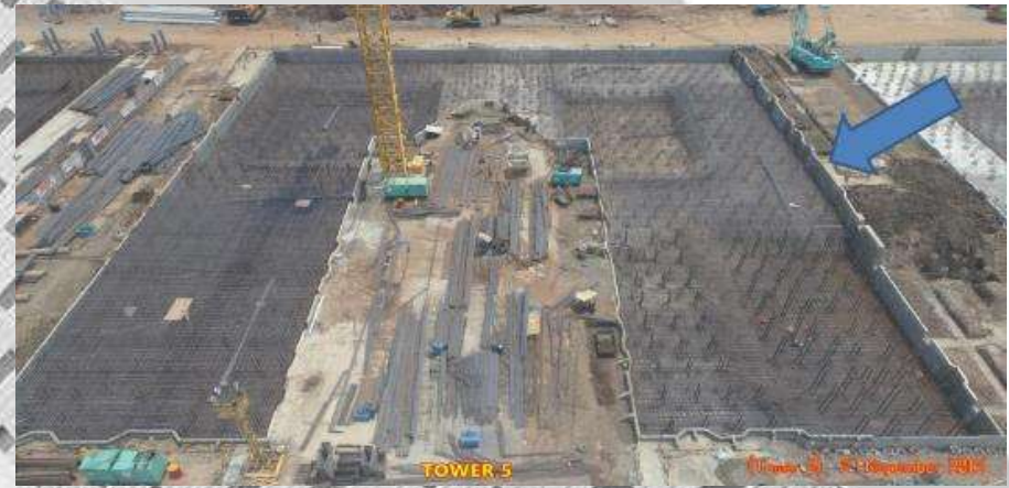
Precast Retaining Wall For Raft Foundation
