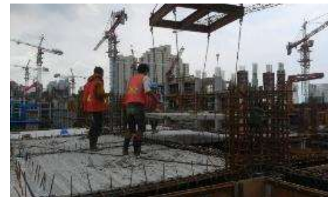
Preslab – Half Slab
