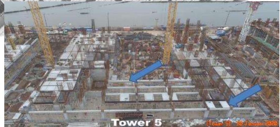
Beam, Half Slab Precast System
