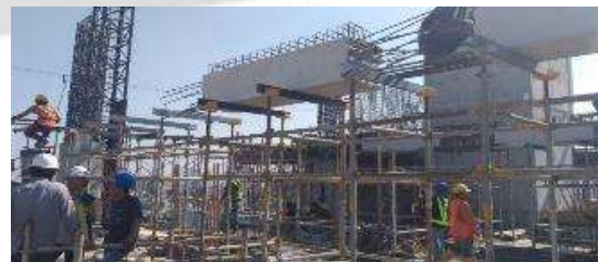
Balok segmental long span dan hollow core slab off site.
